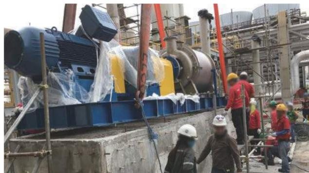
Installation instruction for liquid ring vacuum pump
